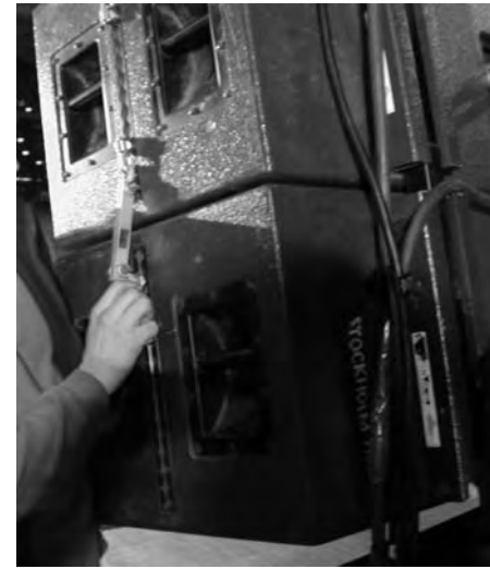
(viii) Connect ANGLE straps on bottom V-DOSC
