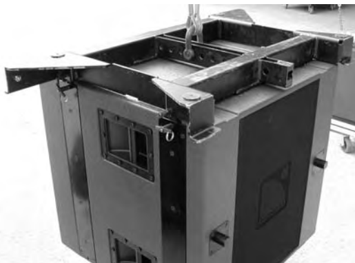
(iii) Fly the first enclosure, pre-attach 4 x dV-ANGLESD, land on the second enclosure, secure using dV-PIN25 then repeat this procedure
