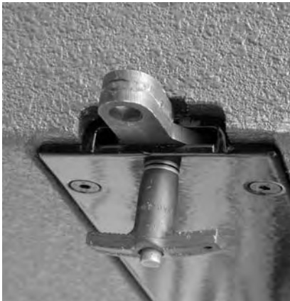
(i) dV-ANGLESD pre-attached - note that the stacked hole position has been selected and the "fat" part of the angle bar is oriented towards the center
