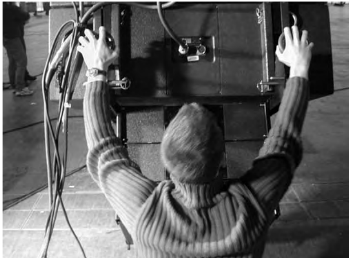
(x) Tighten screwjacks to remove this gap
