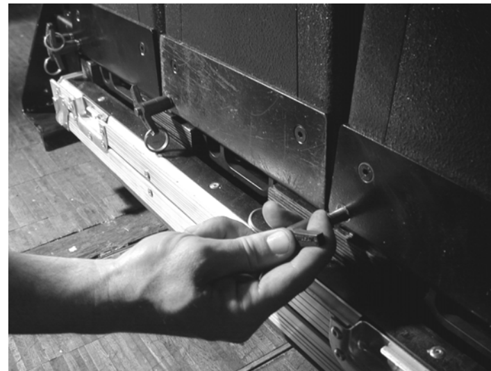
(ii) Pin the fronts of all dV-DOSC using dV-PIN25
